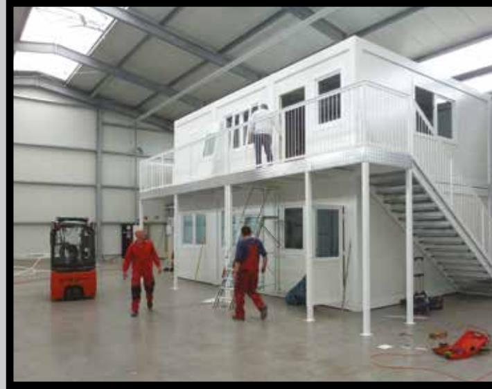
Bureaux - Allemagne Offices - Germany
