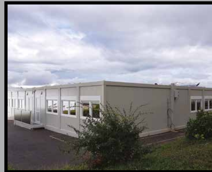
Ecole temporaire - Suisse Temporary School - Switzerland
