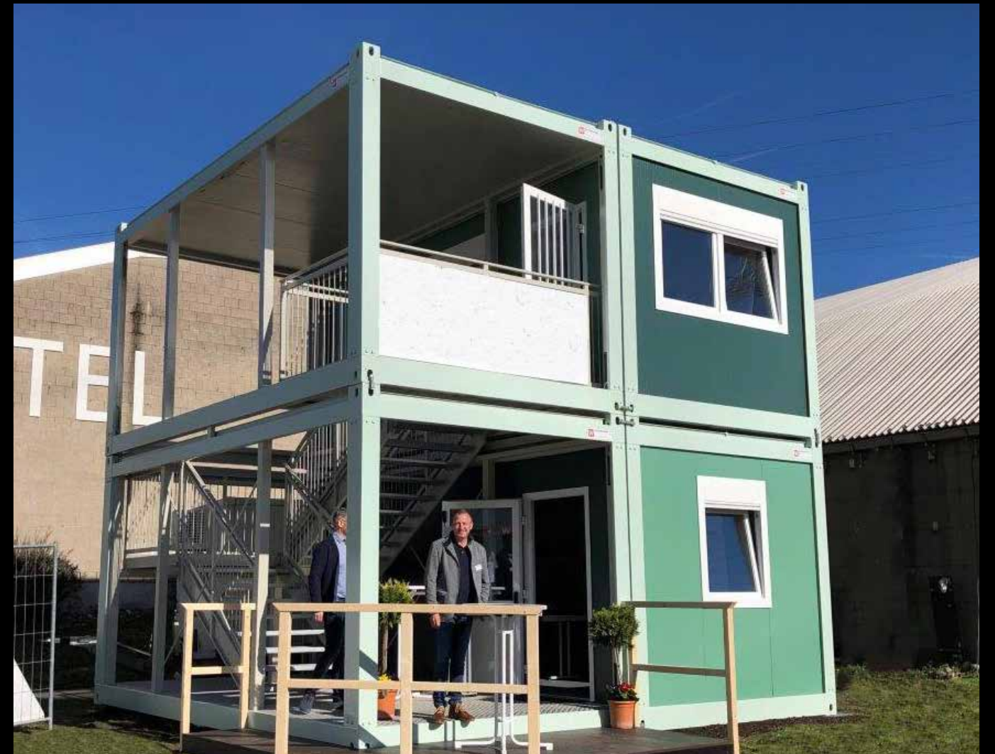
Bureaux - Allemagne Offices - Germany
