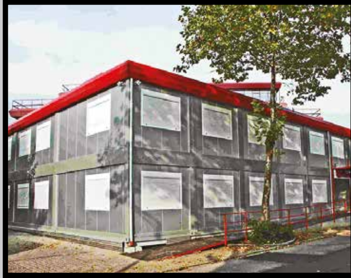
Bureaux - Allemagne Offices - Germany
